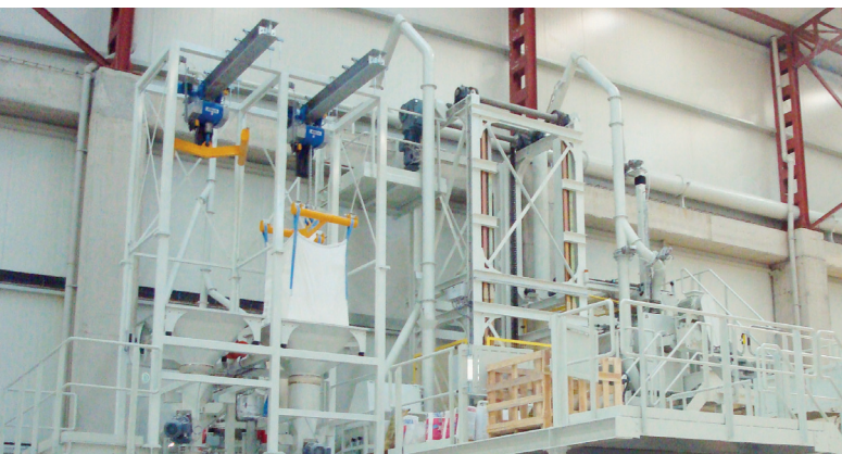
2 Big Bag emptying station in Batchbin system
