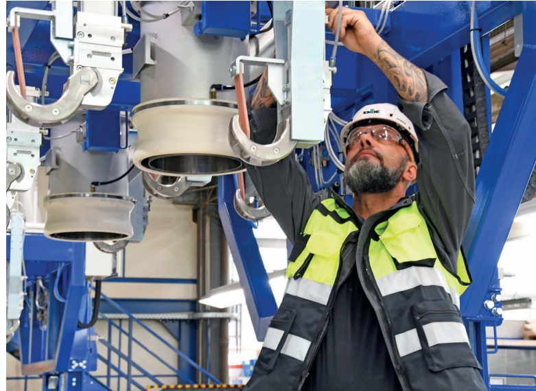
Qualified service technicians
