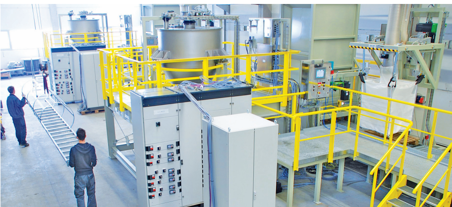
Setting up plant for works approval
