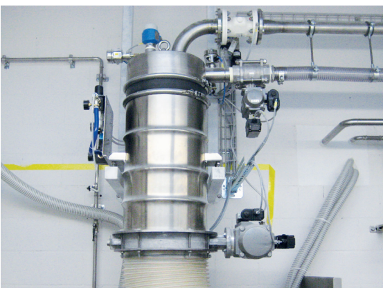
Vacuum conveying for sugar
